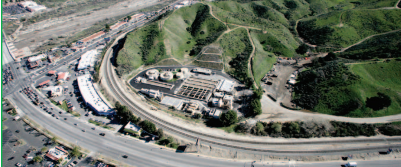
▲ The Sangus Water Reclamation Plant in Santa Clarita, California, cleans 7 million gallons of water per day.
